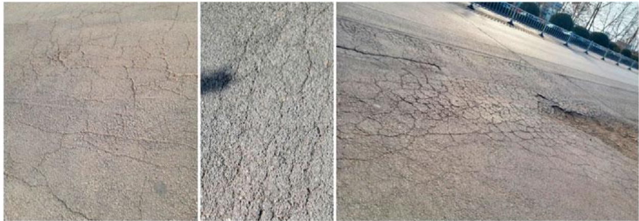
Transverse cracks
