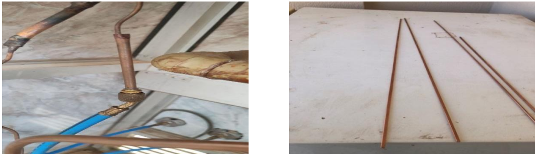
Figure 3 Connection with hoses and silver wires.
